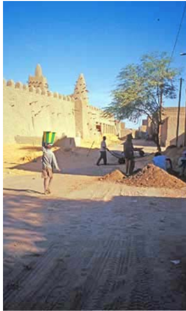
Road work outside the Djingareiber Mosque
