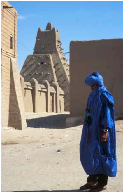
The authors' Tuareg guide and translator, Mohamed Al Hassan Al Ag Moctar dit Halis, stands before the Minaret of the Sankoré mosque. Built of mud plaster, the minaret is pierced with beams that serve as scaffolding when renovations must be done.
